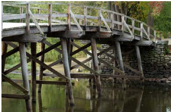
Old North Bridge in Concord, Massachusetts
