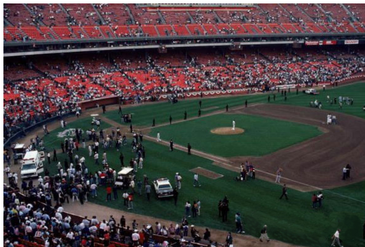
Candlestick Park after the earthquake
