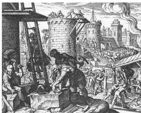
Rebuilding the City
