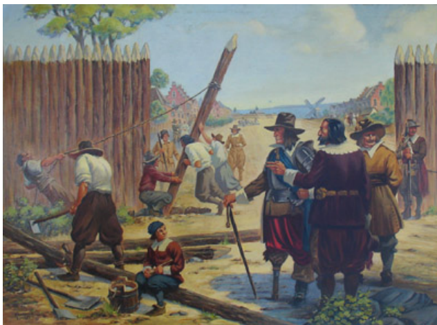
Construction of the Timber Wall at Wall Street, by Frederick Elmiger
